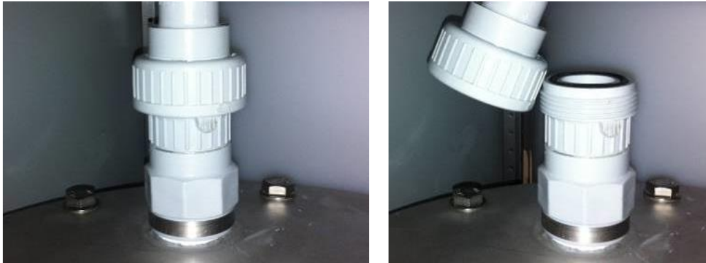
Figure 16: Disconnecting top hose of the resin tank
