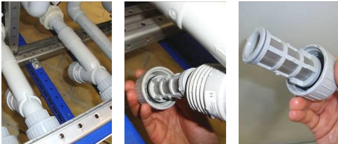
Figure 9: Check on line strainers
