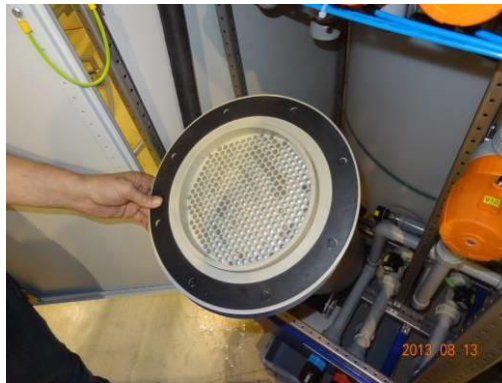
Figure 38: Closing the resin tank after filling up the filter bag and put in the plastic cap with the perforated side down
