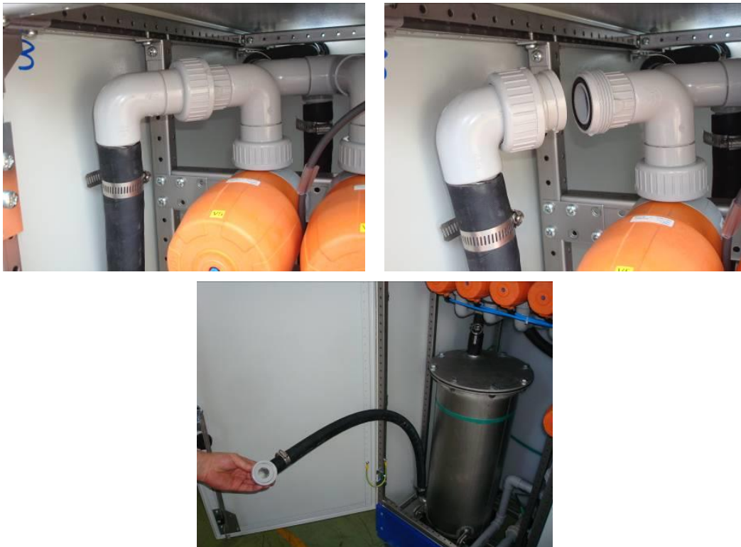
Figure 35: Disconnecting left hose of the resin tank
