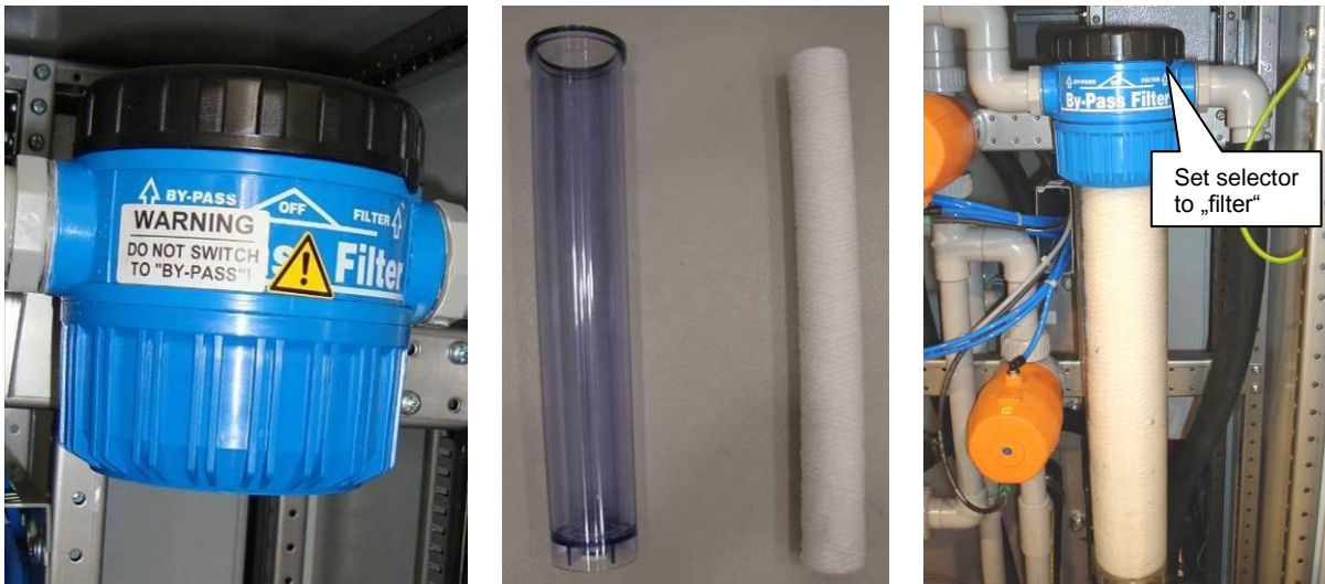
Figure 7: assemble the main filter
