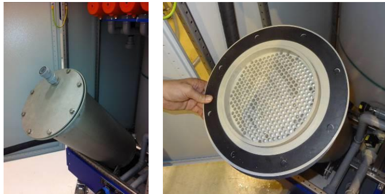
Figure 37: Opening the resin tank
