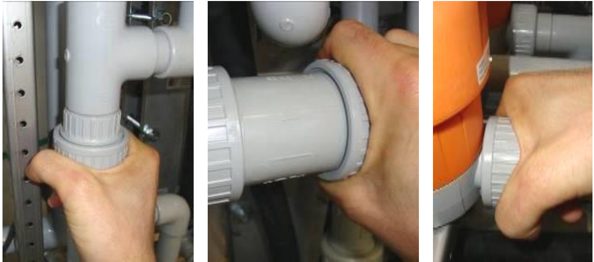
Figure 8: Check union joints on tightness
