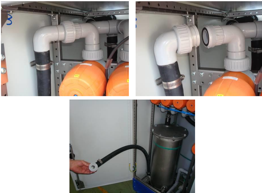
Figure 15: Disconnecting left hose of the resin tank
